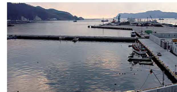
View of Kamaishi Port in Kamaishi, Iwate Prefecture. The restoration of wharfs and seawalls is progressing and the sight of heavy machinery is becoming gradually less common.
